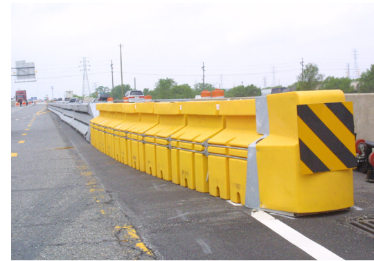
18 Water-filled attenuators for highway collisions give a similar to the concept for the fragments.
